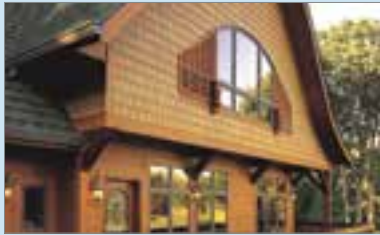
Fiber Cement Siding
