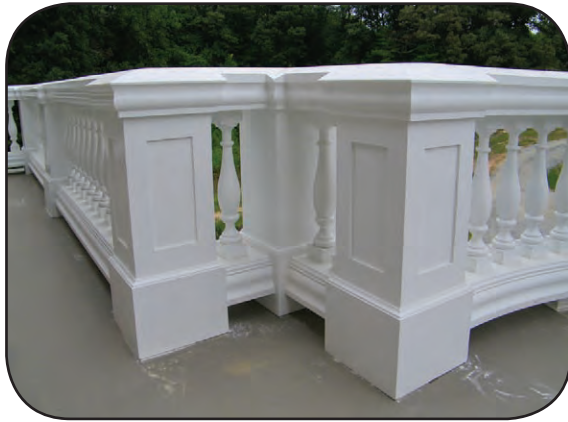
Rail Cap Applique *Coped for fit side of rail.
