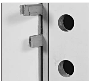
Figure 14: Shims are placed above and below the dead bolt hole (points G in Figure 12).
