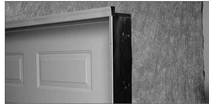
Figure 3: Some door units may be supplied with a plastic skid plate located along the bottom of the door. Do not remove.
