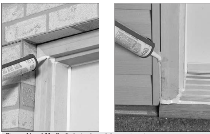
Figures 31 and 32: Caulk the jambs and the exterior trim.
