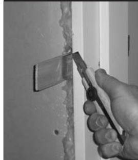
Figure 28: Insulate between the jambs and the wall studs all around the door.
