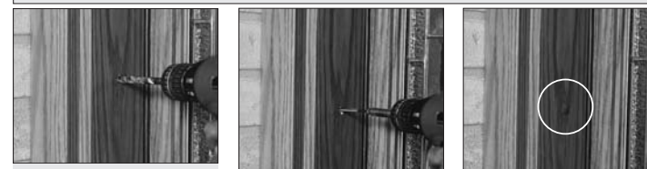
Figure 23: Pre-finished systems must have holes drilled before screws are installed.
