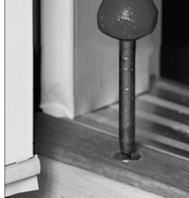
Figure 33: Raise or lower the sill by adjusting the sill screws. Some sills may have covers over the adjusting screws. These covers must be removed prior to making any adjustments.
