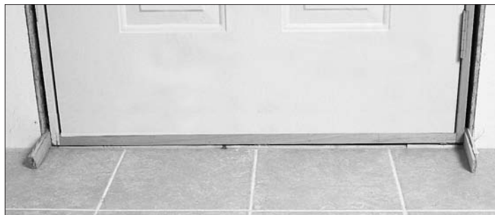
Figure 13: Proper position of shims at the bottom of the door (Points A).
