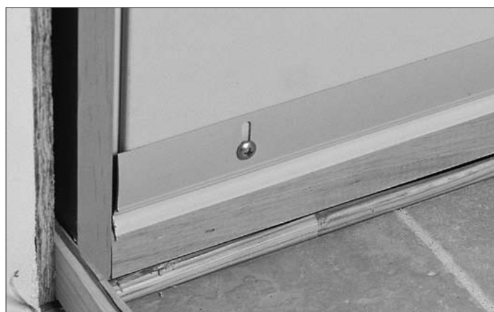
Figure 34: U-channel sweeps are adjusted to form a tight seal with the sill.
