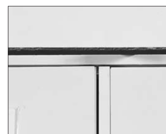
Figure 19: The gap between the door slabs and the head is evenly aligned.
