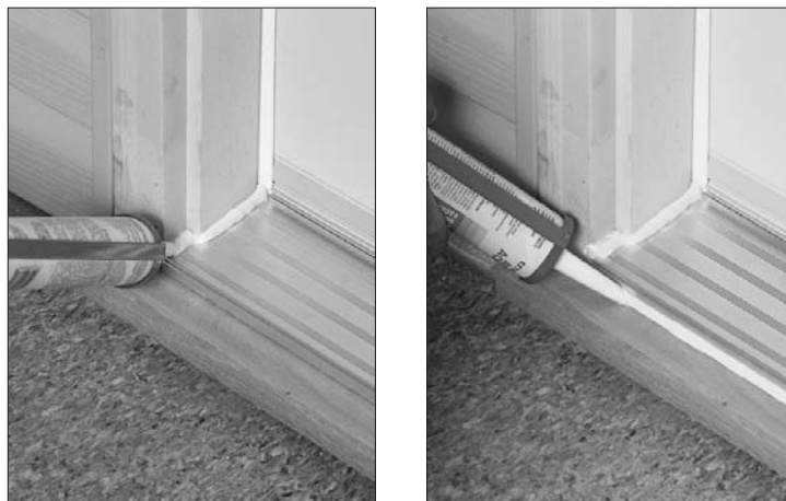
Figures 29 and 30: Caulk the sill crown and the front of the sill.
