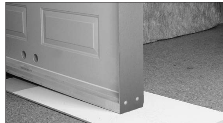
Figure 4: Some door units may be supplied with a wood or cardboard skid plate located along the bottom of the door. Needs to be removed.
